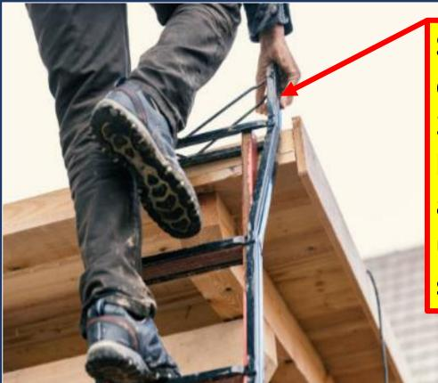
Side rails must extend at least 3ft above the landing if accessing an upper landing such as a roof
